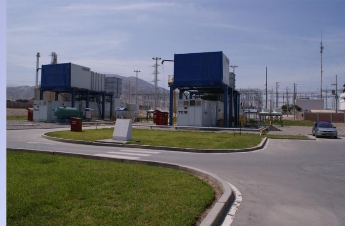
CENTRAL TERMICA PISCO 74.8 MW
