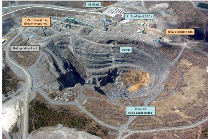
Surface Ventilation Infrastructure (source: Mining Magazine, 2007).
