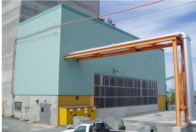
Exterior view of Bulk Air Cooler (source: Mining Magazine, 2007).
